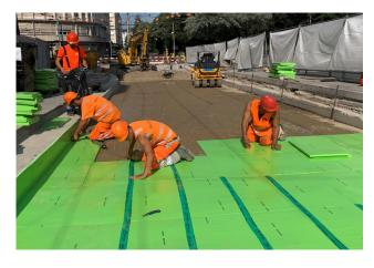
The concrete slab of the tram trough is elastically supported on insulating mats type PURASYS **vi-bra**foam. The mats are laid flush with the level of the substructure or glued vertically to the negative concrete and the shuttering.
