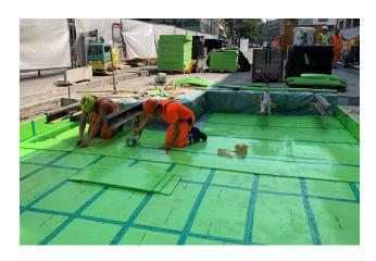
The insulation mats were seamlessly led to the insulation under the existing tram troughs. The stiffness of the mats in the transition area between the new mass-spring system and the exisiting tram troughs was specifically adjusted.
