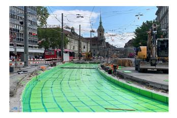
Ready laid horizontal and vertical PURASYS **vibra**foam insulation mats. A protective concrecte was placed on the mats immediately after installation.
