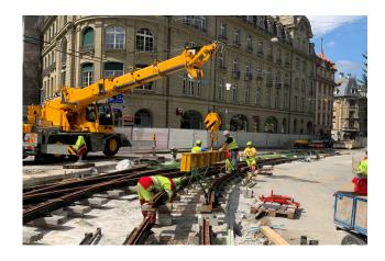
Laying and alignment of the tracks on the protective concrete over the PURASYS **vibra**foam insulation mats. In a next step the tram trough could be concreted out.
