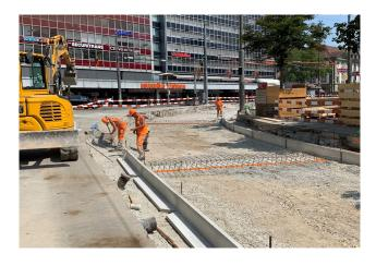
Preparation of the substructure and shuttering. The concrete expansion ledgers for fixing the track trough in the curve area were decoupled with insulating mats of the type PURASYS **vibra**dyn.
